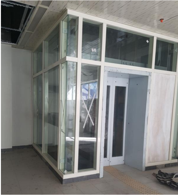
Ongoing Installation of Glass Cladding in Elevators at Emerald Station
