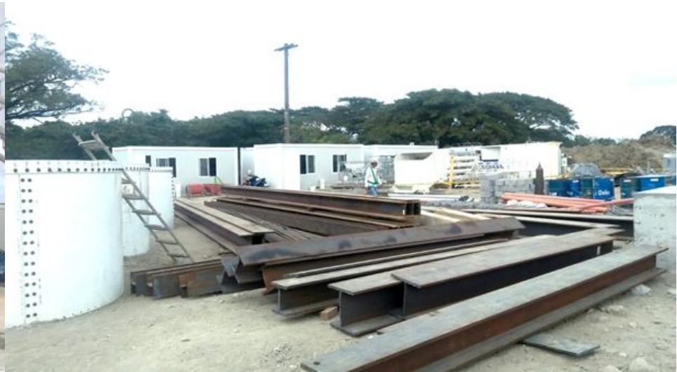
Ongoing Construction of Temporary Site Office at CW 3 Meycauayan Construction Yard (As of 31 January 2020)
