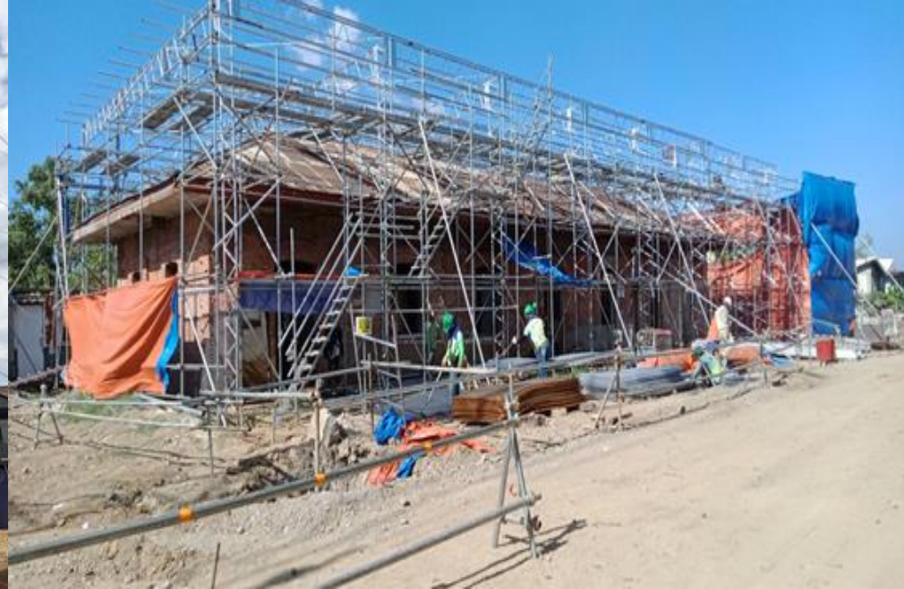
Installation of Protection to Malolos Old Station (As of 22 January 2020)
