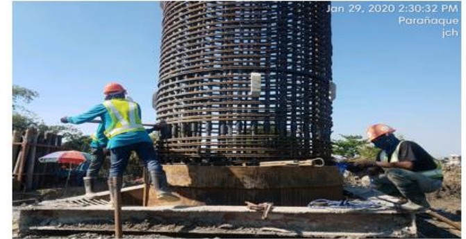
On going Pier Column Works
