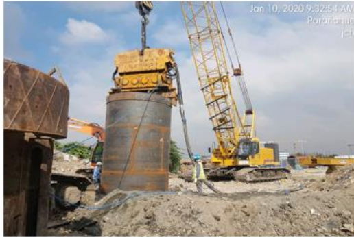
Ongoing Bored Pile Works
