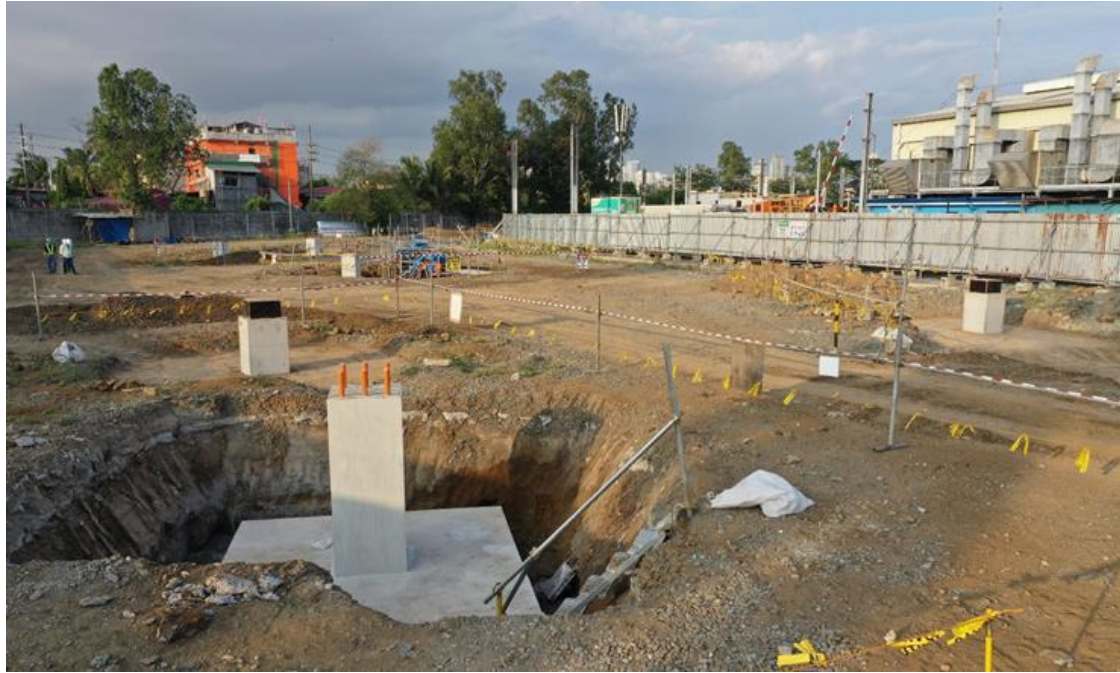
As of January 2020, on-going construction of OCS Foundations
