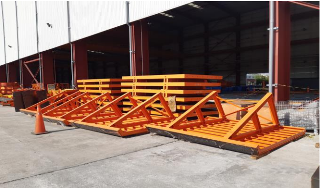
PI Girder Molds was Delivered, Start of Assembly works for PI Girder Molds
