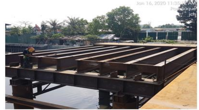
Ongoing installation of steel casing, I-beam framing and deck planks
