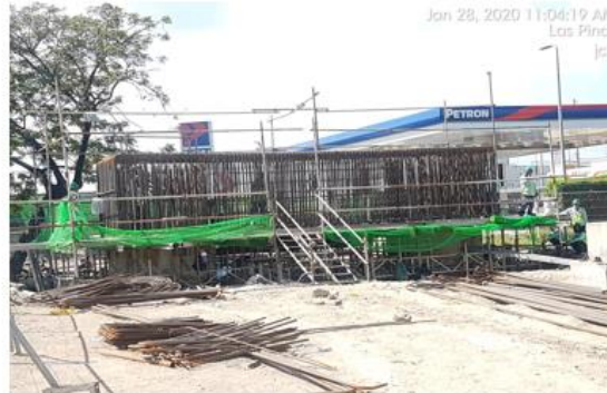
Ongoing installation of pier head / portal beam reinforcement
