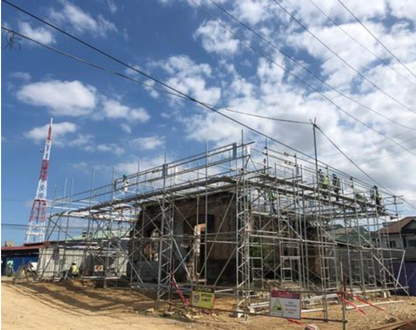
Installation of Protection to Guiguinto Old Station (As of 23 January 2020)
