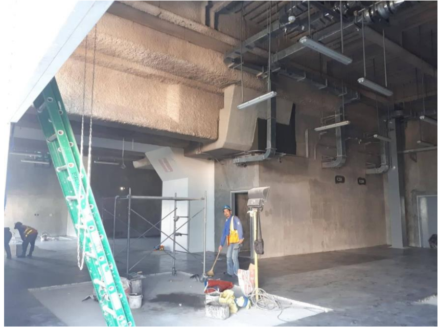
Ongoing Electrical & Mechanical Installation, and Architectural Finishing Works in RSS7 at Masing Station
