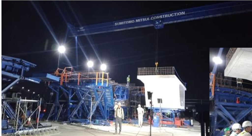
Transferring of 1st Precast Segment to PR 5- 114 to PR 5- 115 (As of 27 January 2020)
