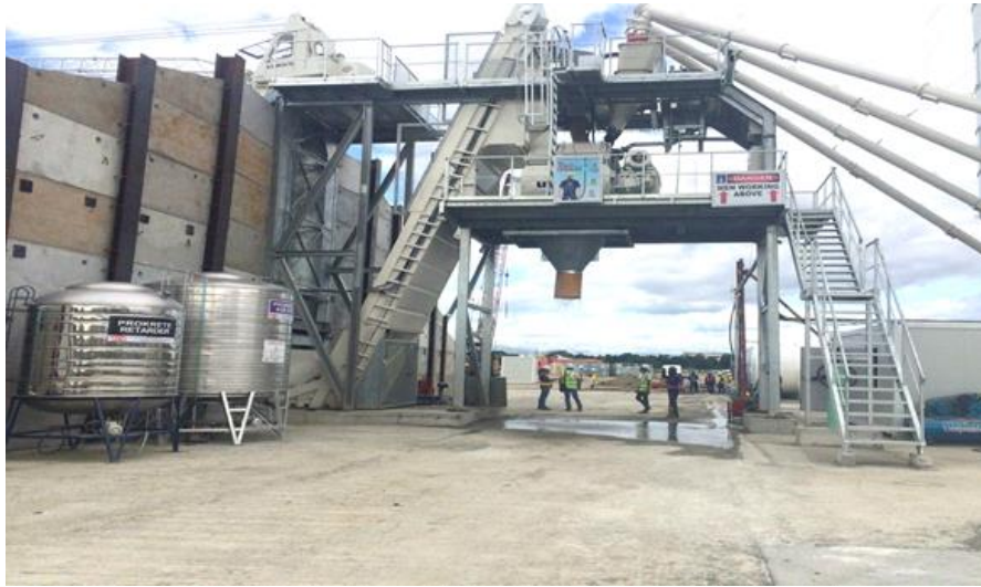
Ongoing Construction of Batching Plant at CW 3 Meycauayan Construction Yard (As of 31 January 2020)
