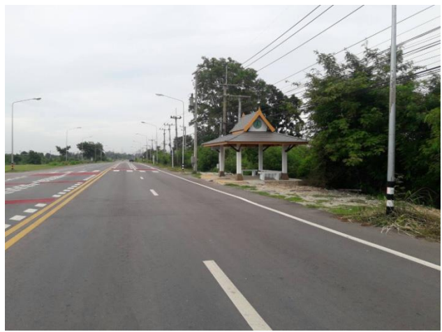
Crosswalk & Street Lighting Bus Stop
