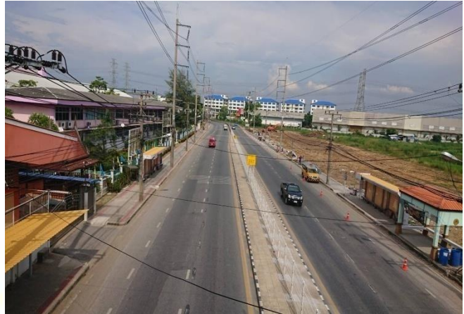
Widening roadway to provide lane for load-unload students
