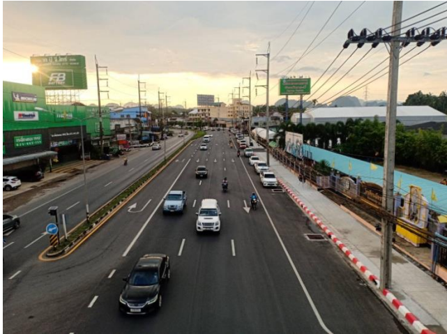
Widening roadway to provide lane for load-unload students
