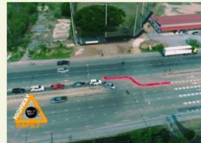
Channelized Lane at Median Opening
