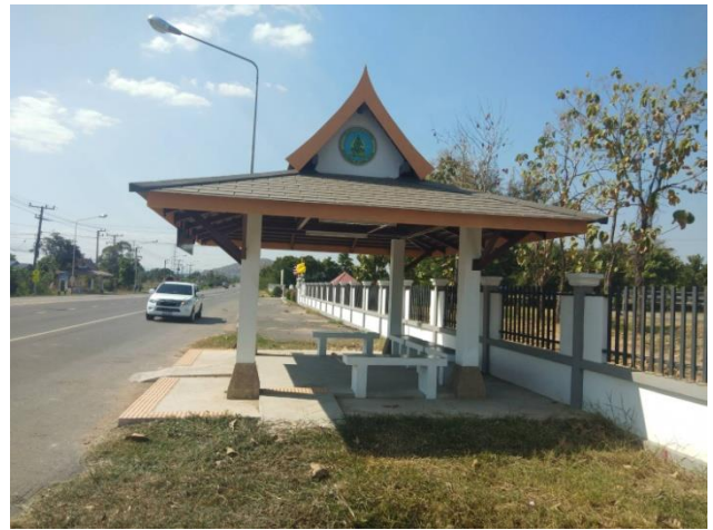
Walkway to Bus Stop Street Lighting
