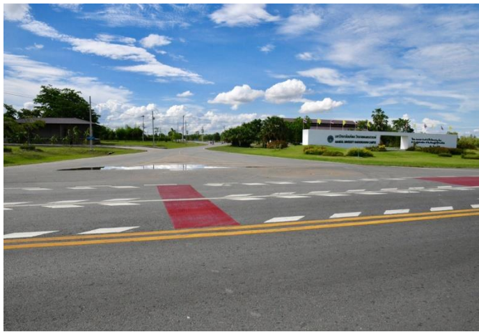
Red Rumble Strips Optical Speed Bar (OSB Marking)
