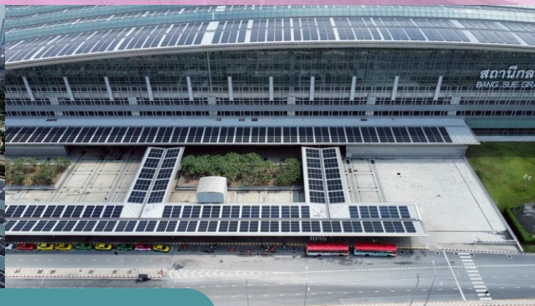
Solar Rooftop Installation
