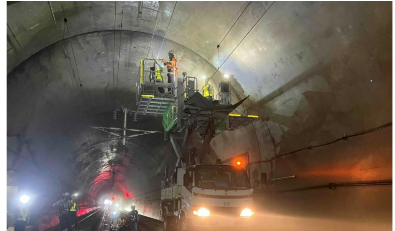
Civil structure (Hammering Test in Tunnel)
