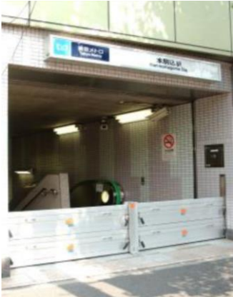
Flood prevention stop boards
