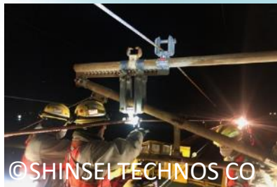
Construction & maintenance works
