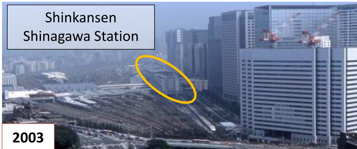
When Shinagawa Station was put in place
