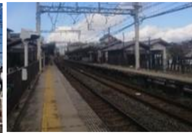
Platform without platform doors
