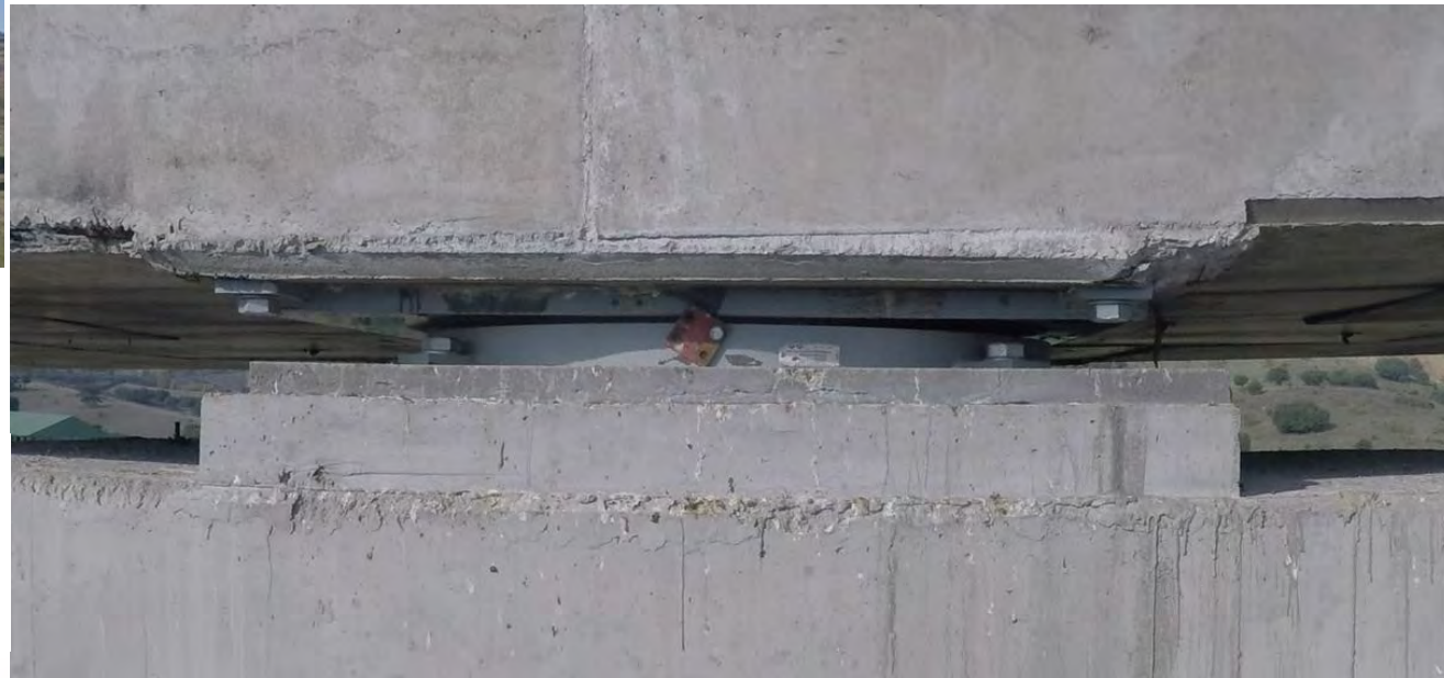
Viaduct in High Speed Line Madrid-Valladolid
