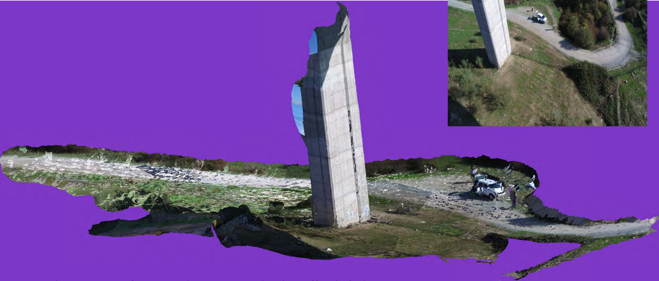
Viaduct in High Speed Line Madrid-Valladolid
