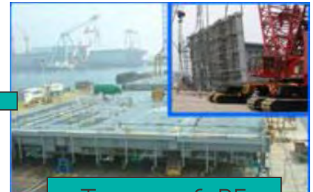
Turnover & PE *Turnover, Outfitting and Pre-erection
