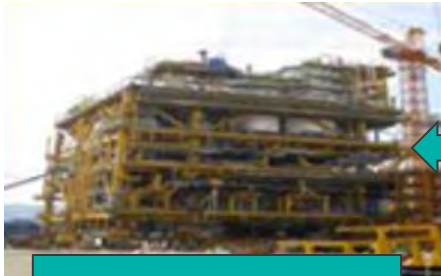
Ready for Lifting
