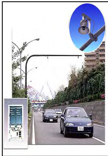
Traffic counters only for traffic signal control
