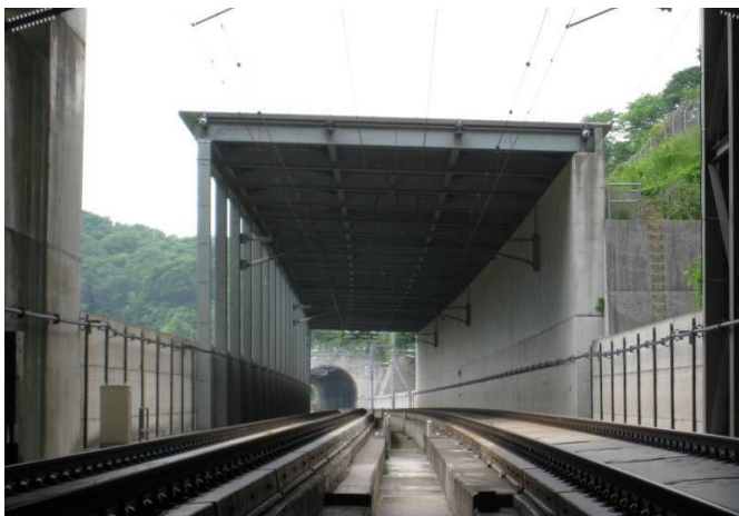
Falling-rock protecting work
