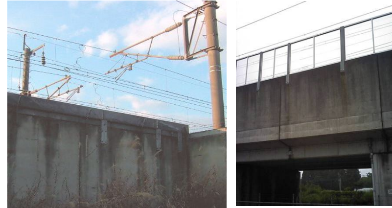
Windbreak wall (Elevated section)
