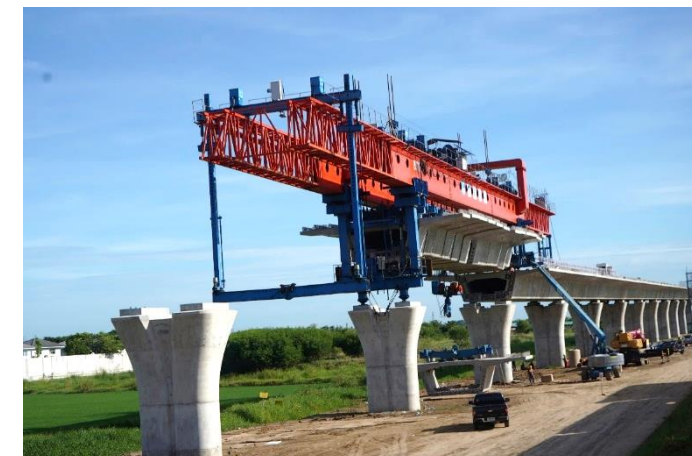
Construction progressing in a elevated section (pictured in July 2023)
