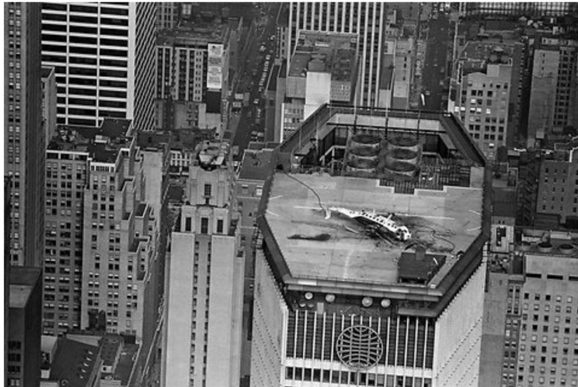
Neal Boenzi/The New York Times The wreckage of the helicopter on the Pan Am Building helipad, which left five people dead on May 16, 1977.
