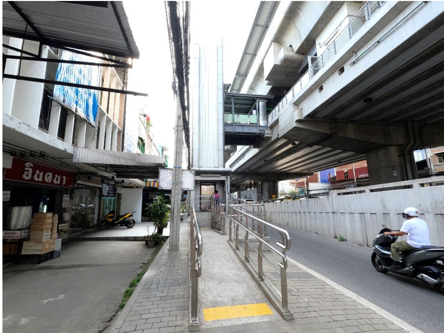
Occupation of a sidewalk by an ancillary facility of a station
