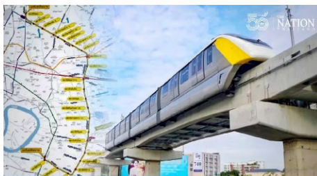
Under construction: Yellow Line
