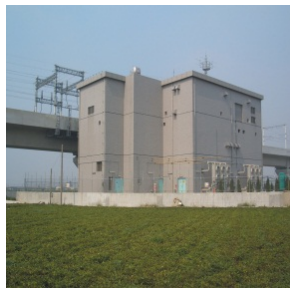
Electric Power Supply
