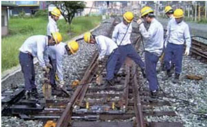
rail track maintenance
